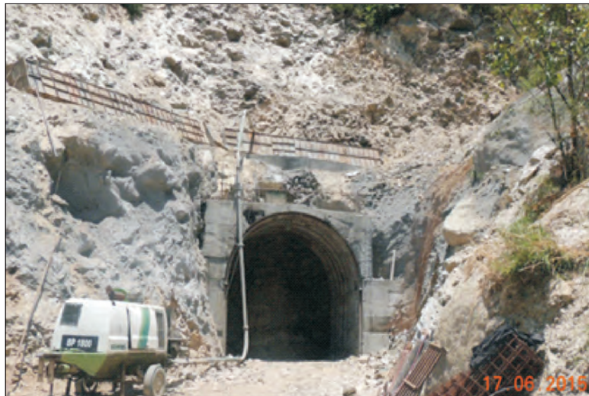
Plate-6: Opening of Additional Adit at Sawra-kuddu HE Project to speed up the HRT Excavation work
