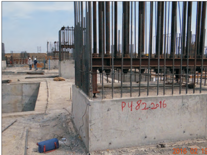
Plate-4: Monitoring of vibration on the close-by concrete structures
