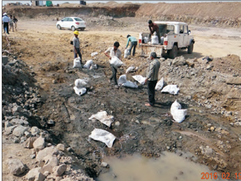
Plate-3: Controlled blasting at 2 x 660 MW STPP Khargone, NTPC, MP
