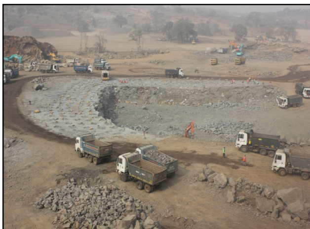
Figure: View of Ulwe Hill site and controlled blasting practices for the flattening of the hill for construction of Navi Mumbai International Airport
