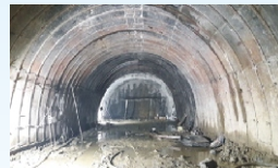
Saranda new railway tunnel in Mumbai-Howrah Railway Line (RVNL)
